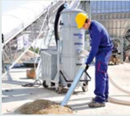
Recovery of high quantity of heavy materials
